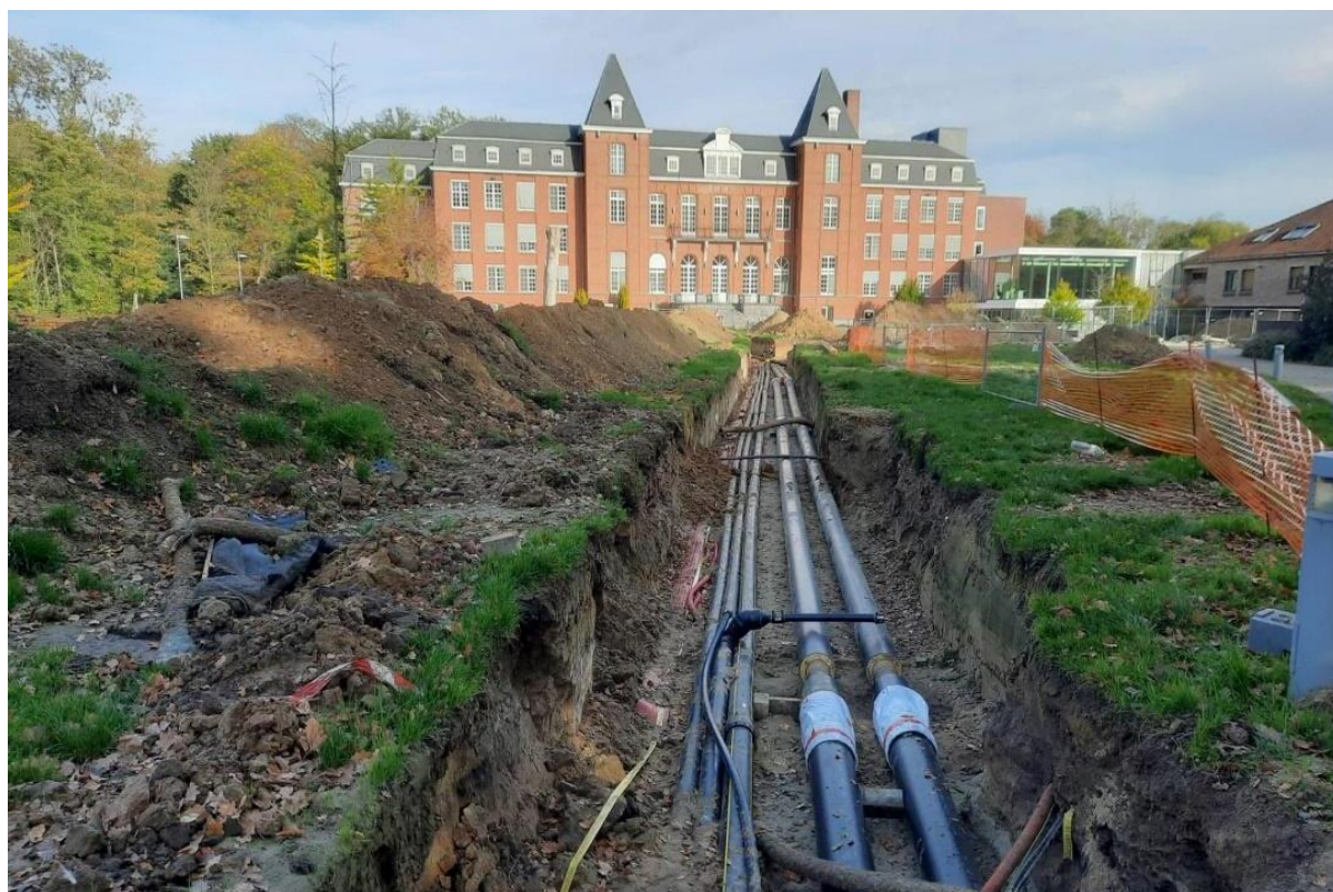
Image 8 - District heating network construction © Beauvent, 2022
